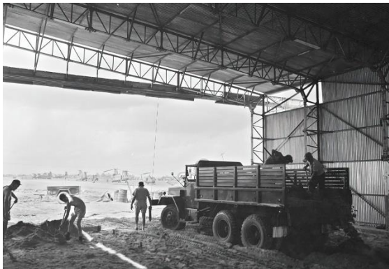
No. 5 Airfield Construction Squadron prepare a hangar floor in Vietnam for the laying of cement. Source: Australian War Memorial
